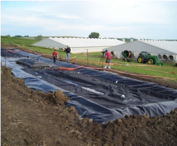
Preparation prior to filling of two bags
