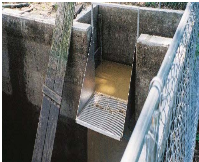
Photographs show (left) cleaning lift station and (right) newly installed self-cleaning screen.
