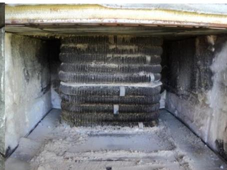
Heat exchanger surfaces fouling with particulate matter
