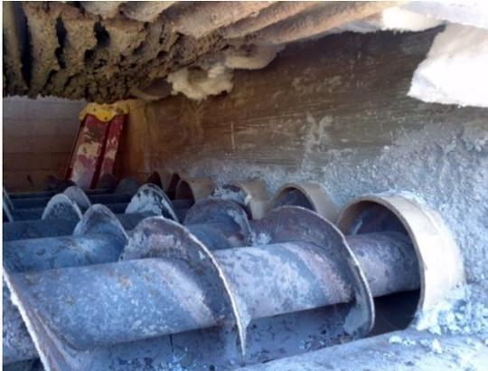
Picture above showing ash bridge or air lock installed with cast refractory
