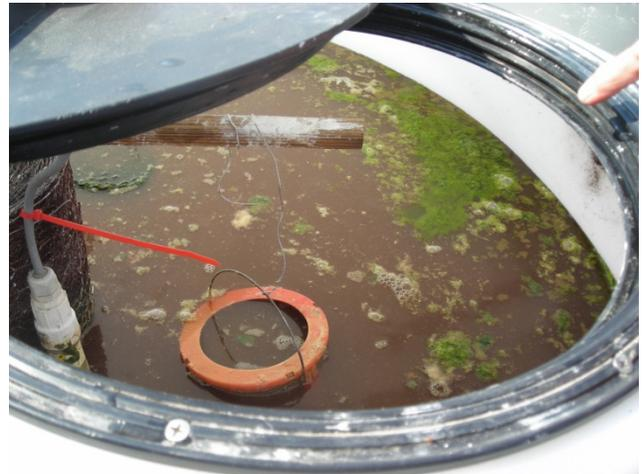
View of inside tanks where chemicals are put in a small basket (round orange ring) and diluted into the effluent batch.
