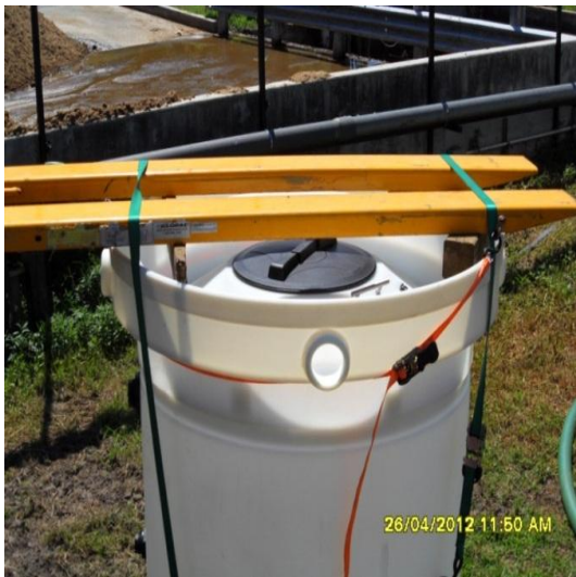
Preparing to lift New Tank.
