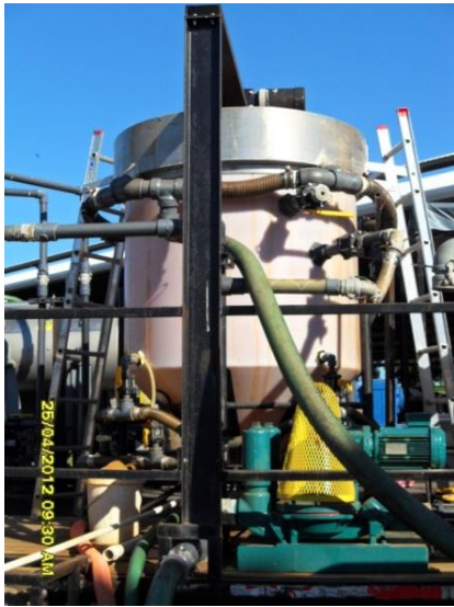
Before removal of 52 in tank
