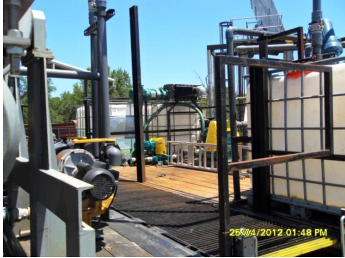
Tank & Frame removed.
